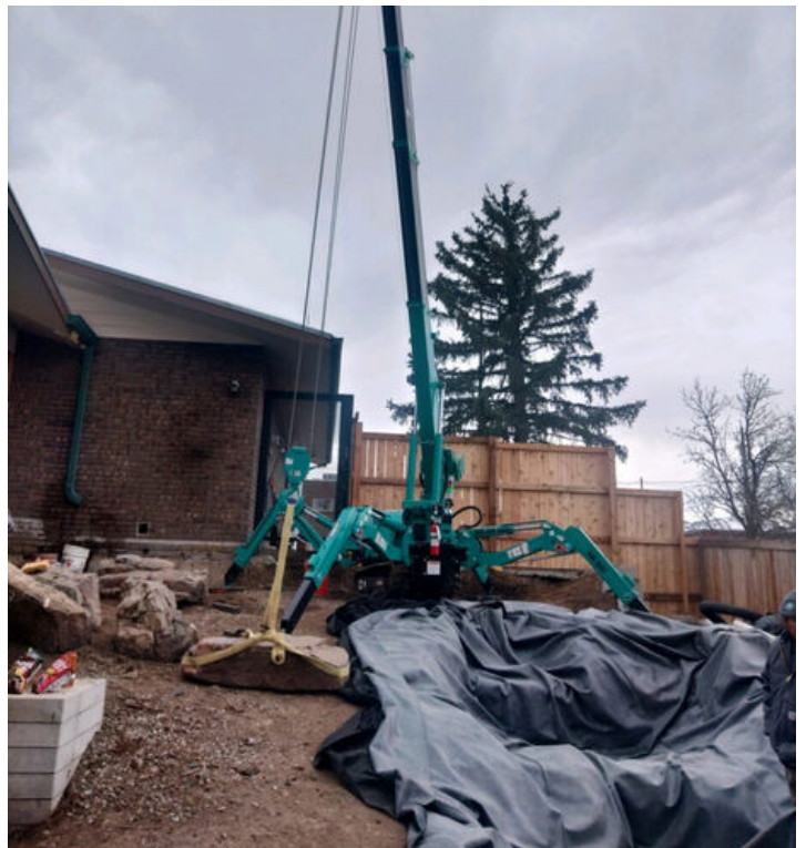
LUXESCAPES SETTING BOULDERS WITH THE SUPERCRANE™ 285 AND WATER FEATURE INSTALLATION FOR A CUSTOMER. WITH LIMITED ACCESS ONSITE, THE SUPERCRANE™ 285 IS WELL SUITED FOR JOBS LIKE THESE.
