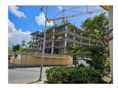
To address these unique logistical demands, Preston Rentals supplied three SuperDeck® platforms: 1 x SuperDeck® 2.6 and 2 x SuperDeck® 3.2s. These platforms offer unmatched versatility, enabling the safe and efficient loading of diverse building materials, including glass, concrete, and mechanical equipment, directly into the structure. Additionally, the decks provide vital on-site storage space, further streamlining the workflow.
